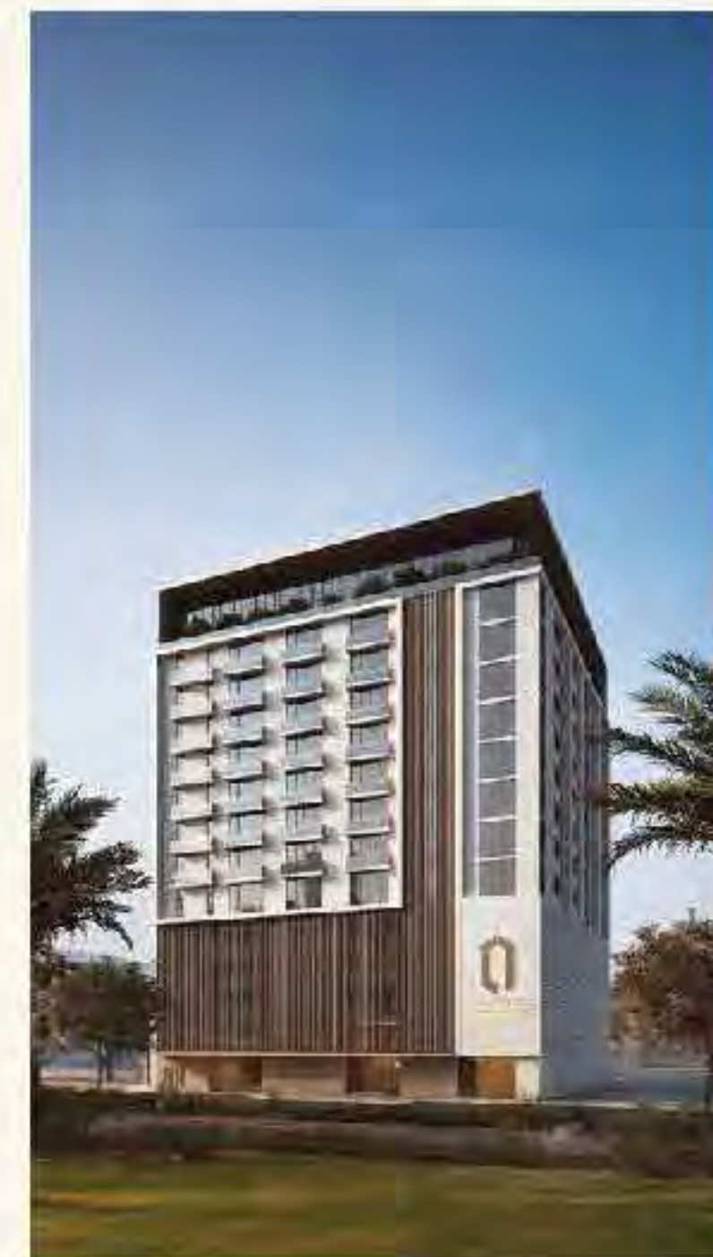
CONCEPT 7 RESIDENCES UNDER CONSTRUCTION
